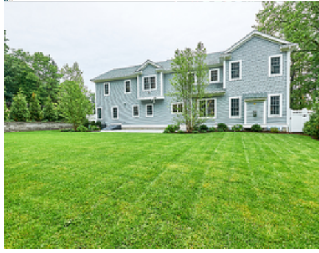
Back Exterior and Yard
