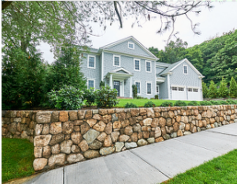
Natural Stone Wall – Front
