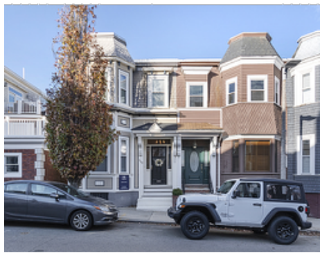
Front View – 520 East 5th Street
