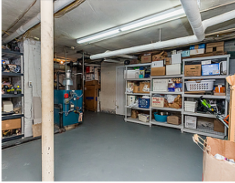
Utilities and Storage
