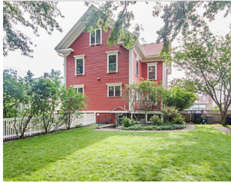
Walk Out Basement
