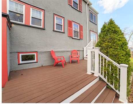
Deeded Side Deck
