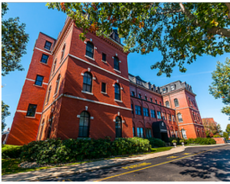
100 Captain's Row Historic Building ~ 1840s
